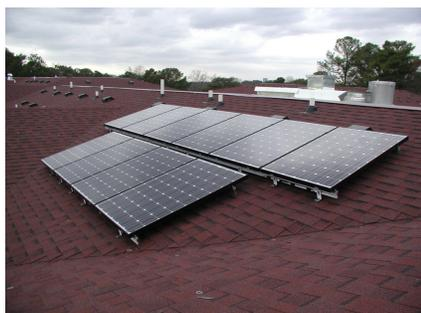
An example of a 2kW array of PV
